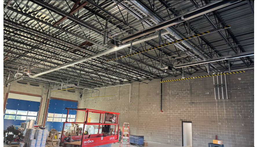
Area C Ceiling Grid/Paint
