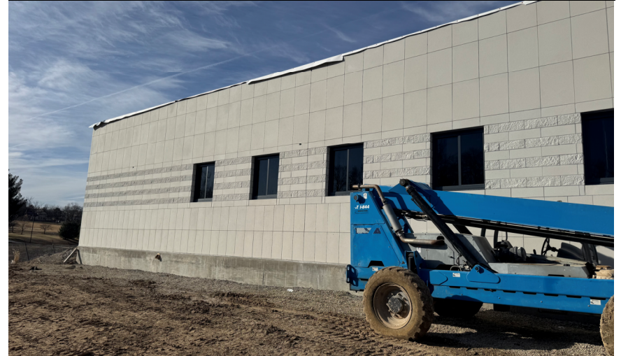
Area A Stone Veneer (Final Section)
