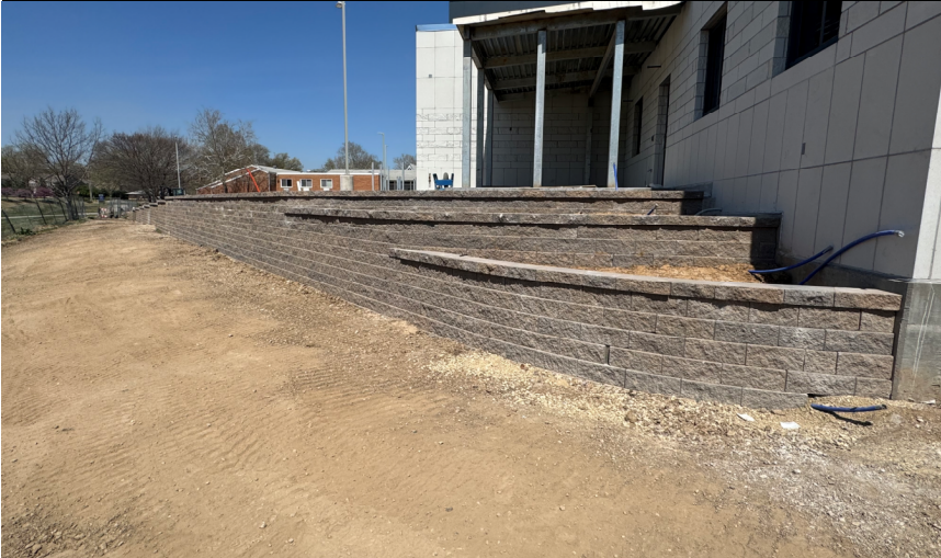
Exterior Retaining Wall
