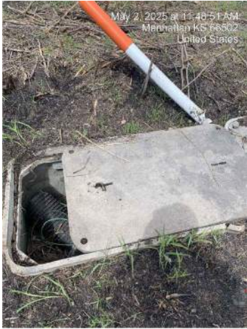
DAMAGED HANDHOLE 1 4
