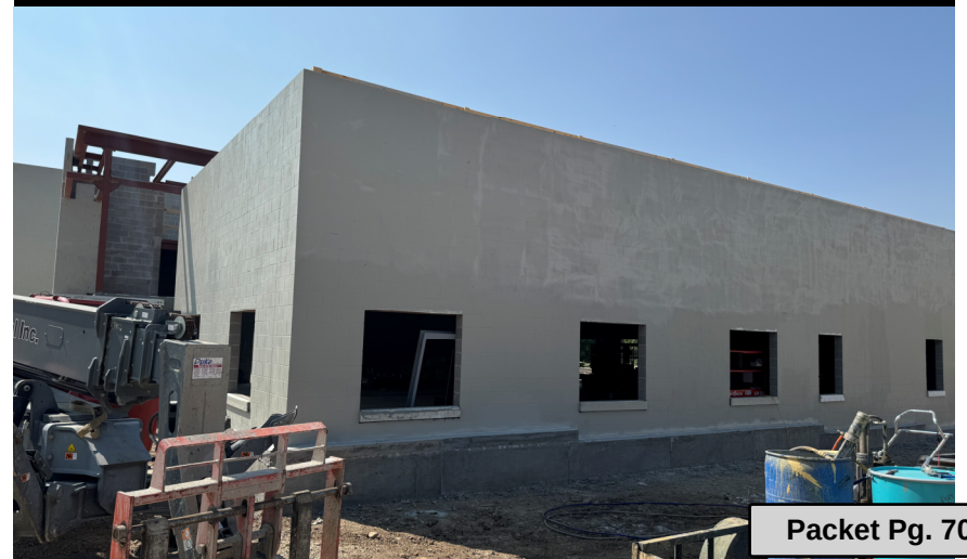
Area C Liquid Water Membrane
