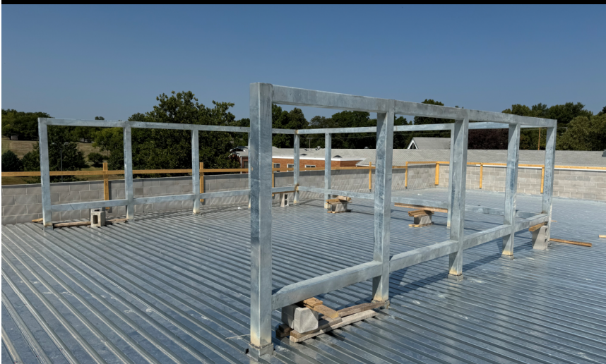
Area C Mechanical Screen Wall
