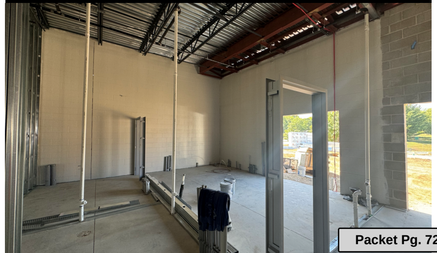
Area C Block Filler/Prime in Mechanical/IT Room
