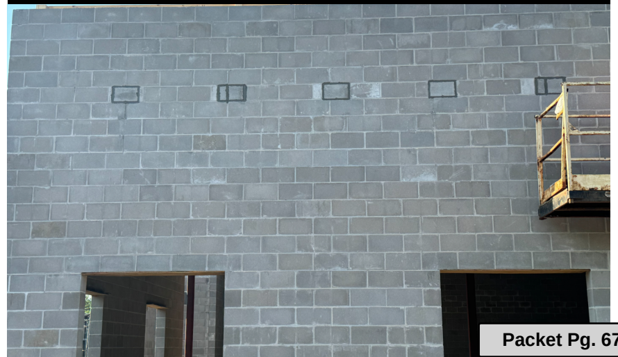
Area C Beam/Joist Pockets
