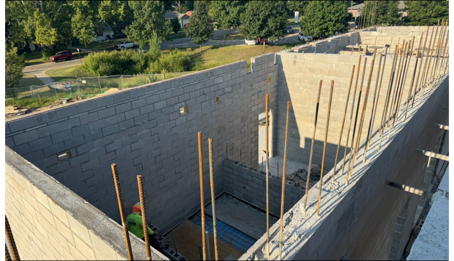
Area C Beam/Joist Pockets
