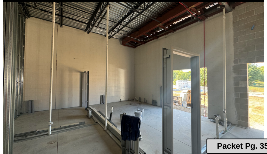
Area C Block Filler/Prime in Mechanical/IT Room
