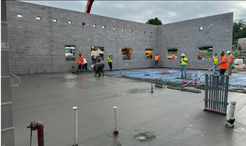
August 6, 2024—Office Area Concrete Slab
