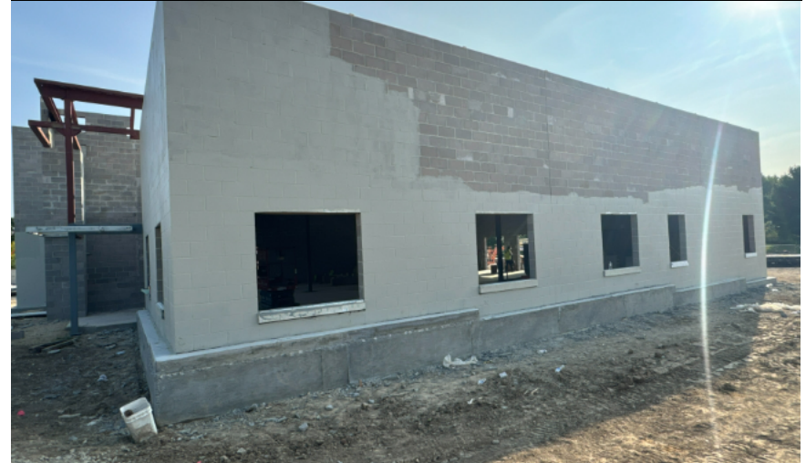
September 10, 2024—Masonry Waterproofing
