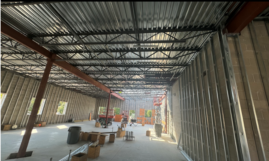
Area A Hanger rough-in for Plumbing
